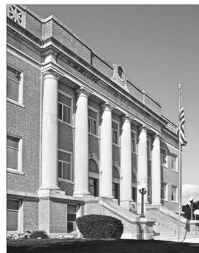
Cheyenne County Courthouse
